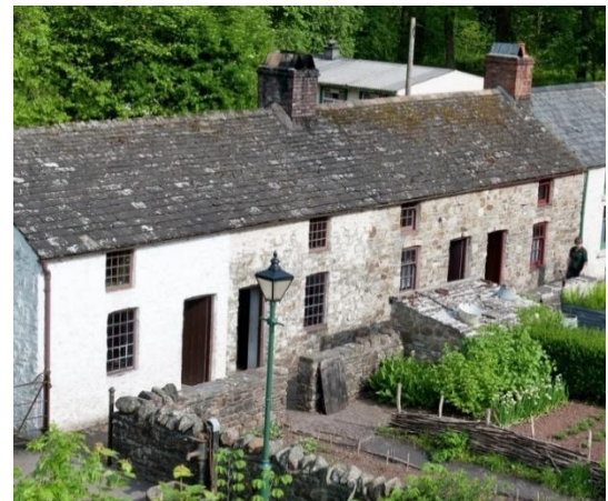
Figure 3. View of Roof Coverings
