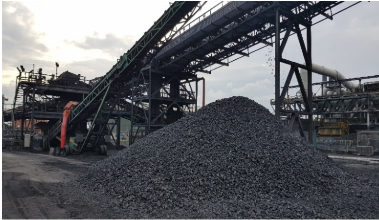
Figure 27 – Coke Stockpile after stacker at Morfa Coke Ovens (Waters, 2018)
