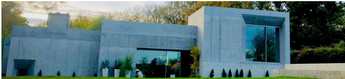
Figure 3: The Concrete House, view of the front elevation
