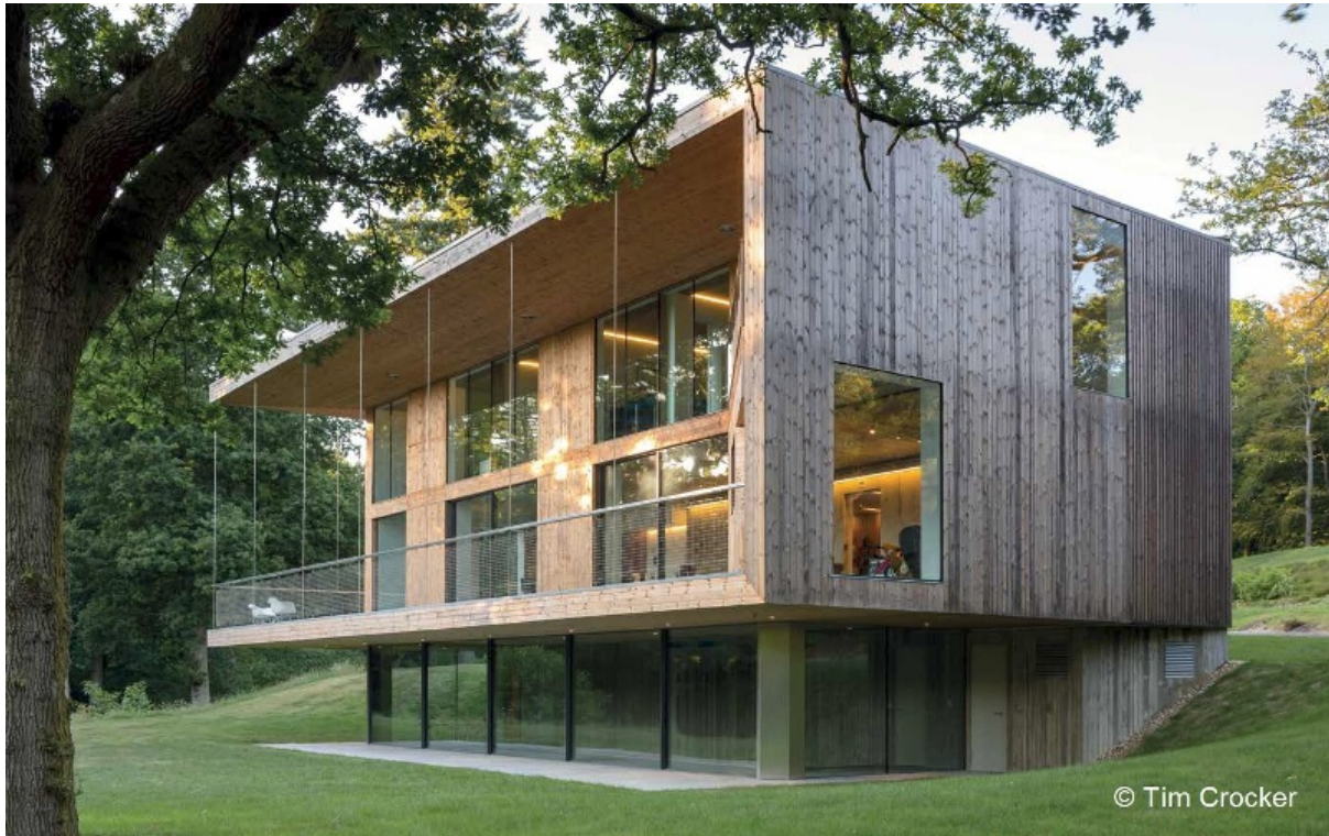
Figure 1: Rear elevation view of the Red Bridge House, Crowborough
