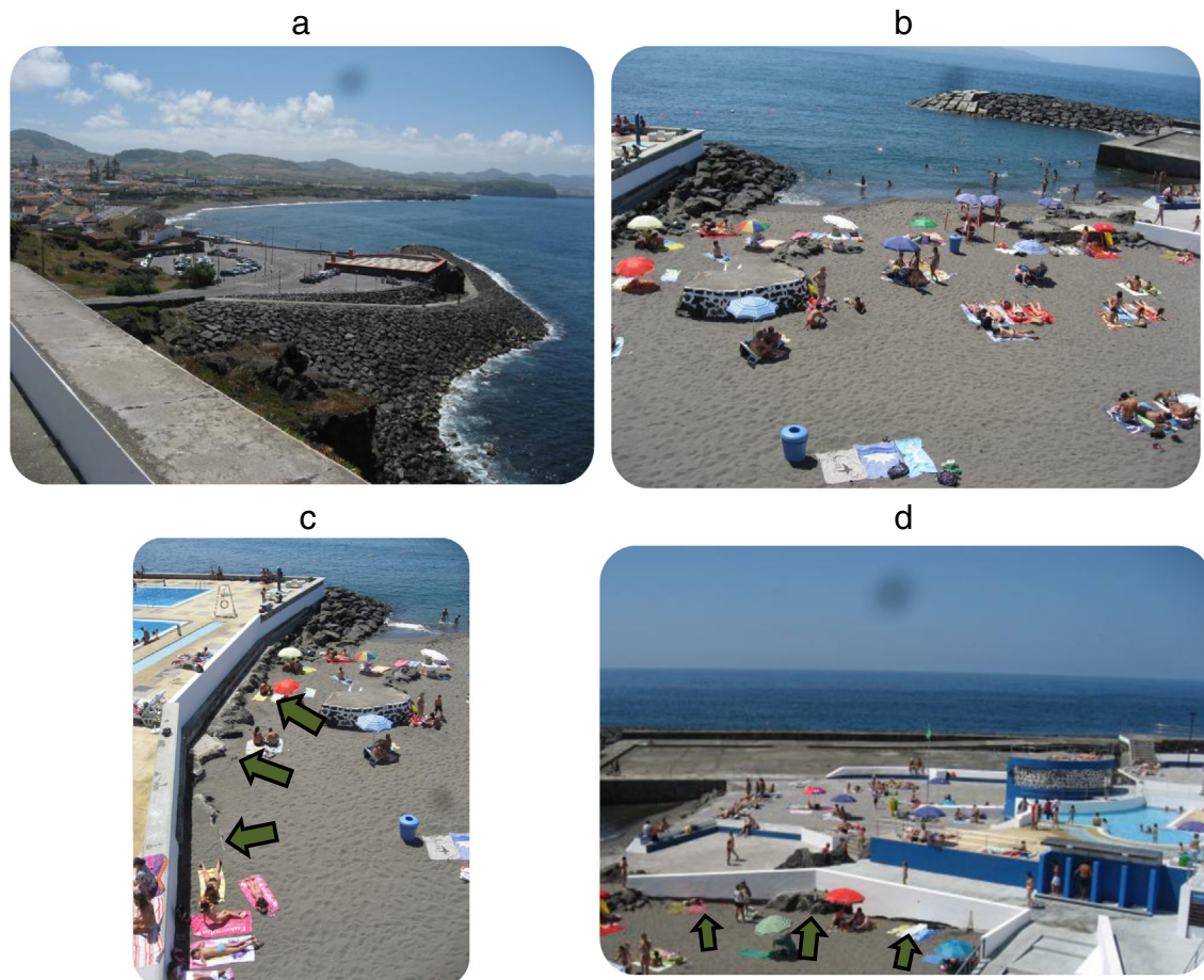
Fig. 11. Ribeira Grande: a) coastal engineering work at Ribeira Grande; b) pocket beach; c) exposed rocks and left-side wall (arrows) and d) exposed rocks and right-side wall (arrows).
