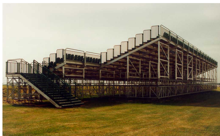
One type of temporary demountable grandstand
