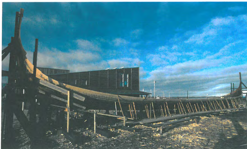
Fig. 1.41. Bottom planking has been mounted to keel and stems, with temporary support from underneath. Photo: W. Karrasch.
