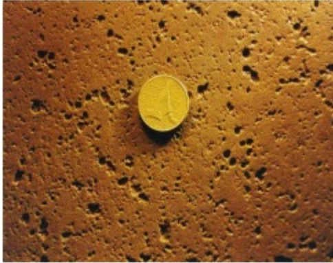
Figure 2: Pits on Metal Surface (Pessu, 2015)
