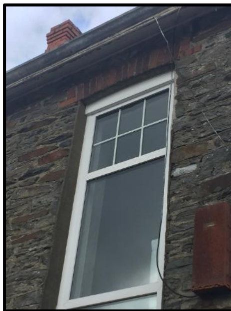
Figure 18 = Concrete & Brick Lintels above windows on right side of building. Giles, 2019
