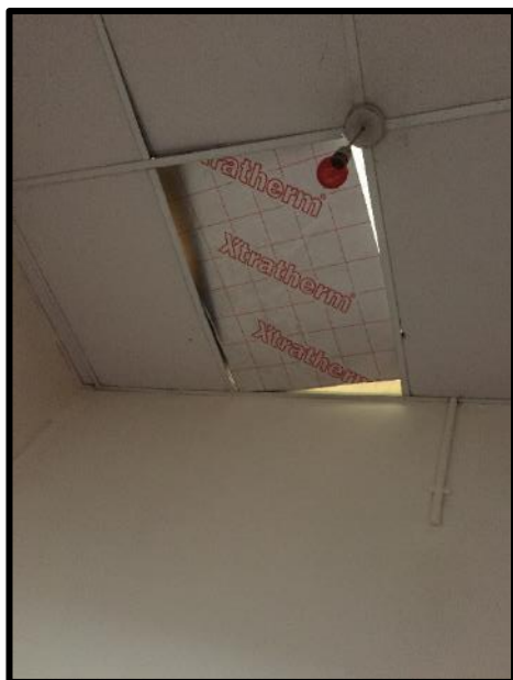
Figure 22 = Loose ceiling in lobby and stairs to first-floor. Giles, 2019
