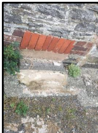
Figure 19 = Doors and filled in coal bunker on right side of building. Giles, 2019
