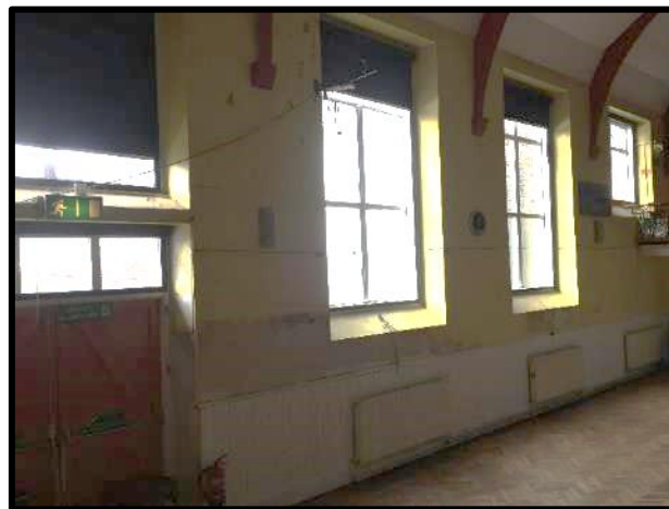
Figure 30 = Main Hall Windows & Double Door. Giles, 2019
