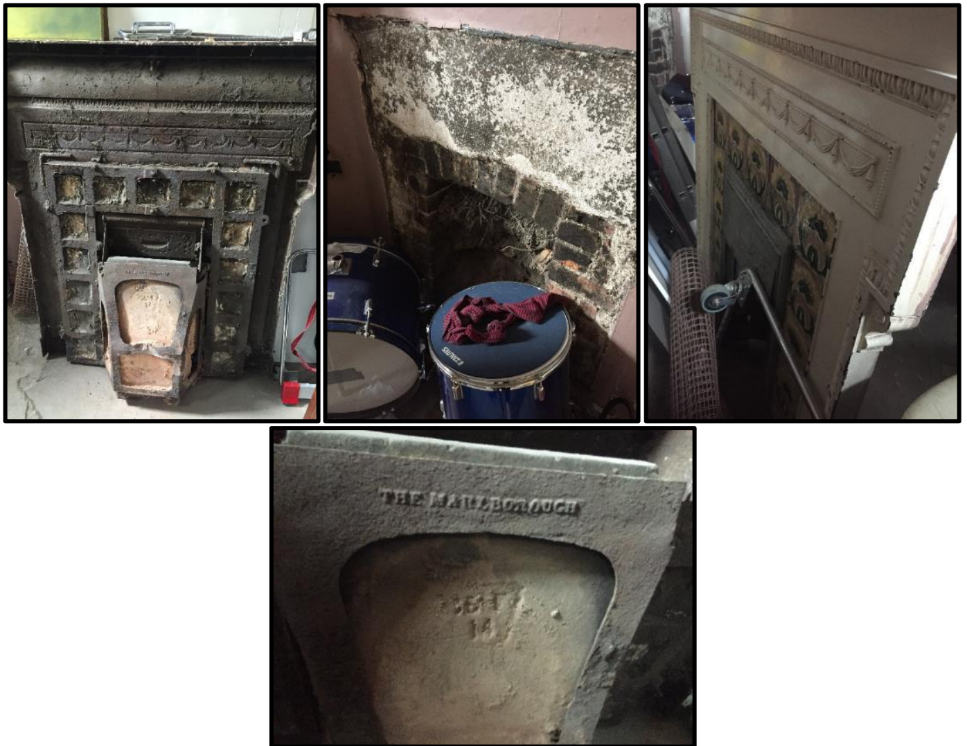
Figure 34 = Marlborough Fireplace in Green Room Stage Right. Giles, 2019
