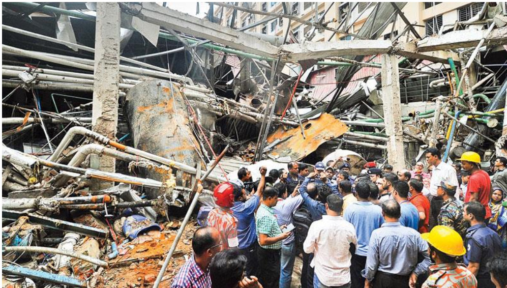
Figure 7. Catastrophic failure of a shell boiler, Gazipur, Bangladesh (Muhmud, 2017)
