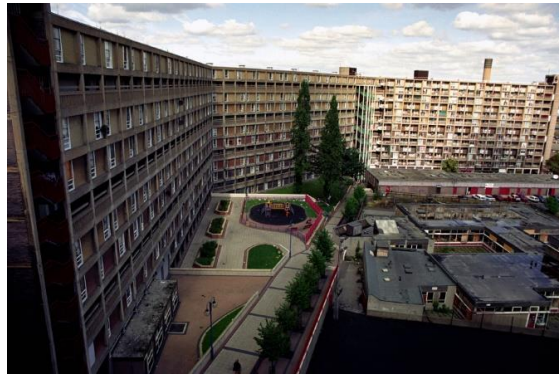
Image 1. Park Hill estate before it was renovated
