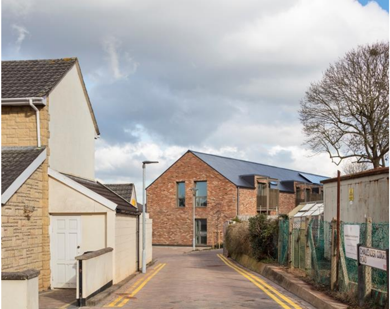
Figure 6 Image of Challender Court (Photo credit Craig Auckland)
