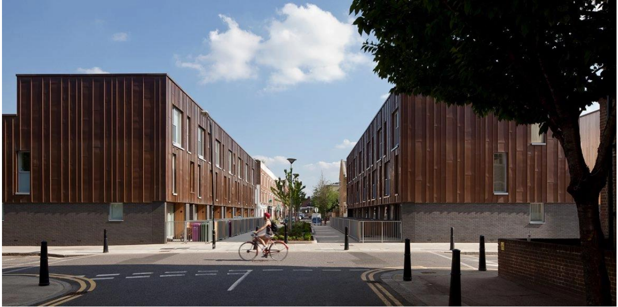
Figure 14 photo of Claredale Street (Photo Credit Tim Crocker)
