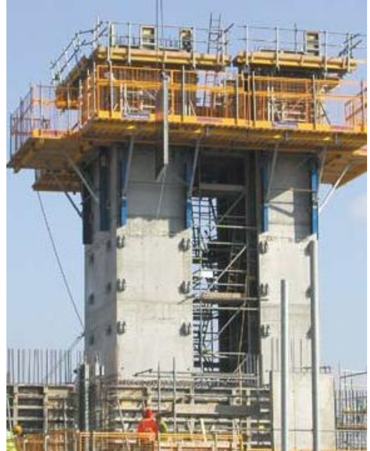
Climbing formwork London, Dorka
