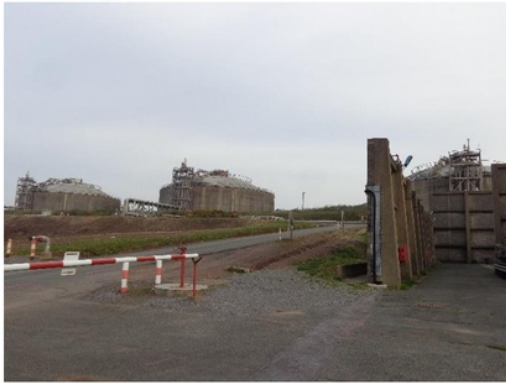
FIGURE 1 - TANK 831, TANK 832 AND TANK 833
