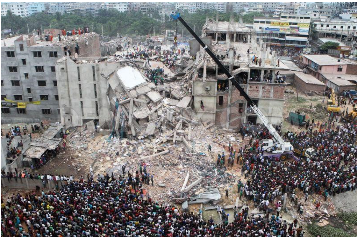
Fig 3: Rana Plaza collapse
