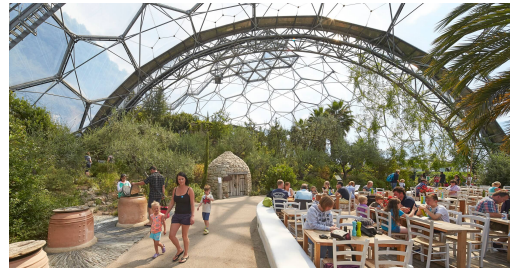
(Figure 12) Internal image of the Eden Project biomes. Image shows the large cladding panels. (Grimshaw Architects, 2021)
