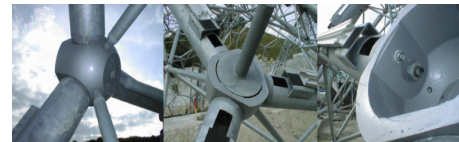
(Figure 9) Node point connection. (Knebel, Sanchez and Zimmermann, 2001)
