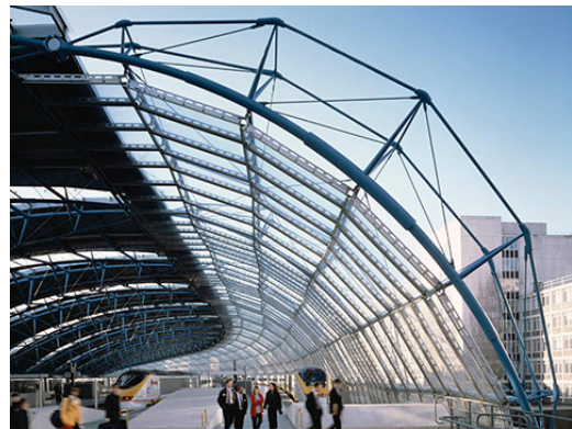
(Figure 3) Roof structure of Waterloo Station. (Grimshaw Architects, 2021)
