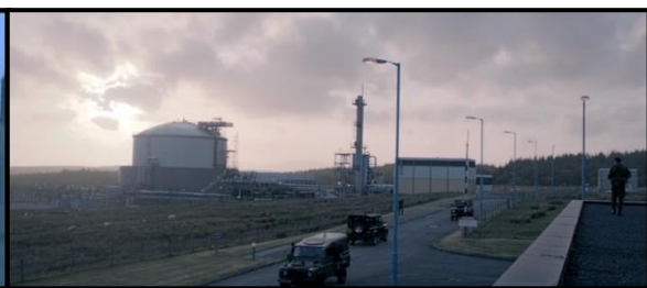
Figure 2. Baskerville Research Facility (Gatiss, 2012)
