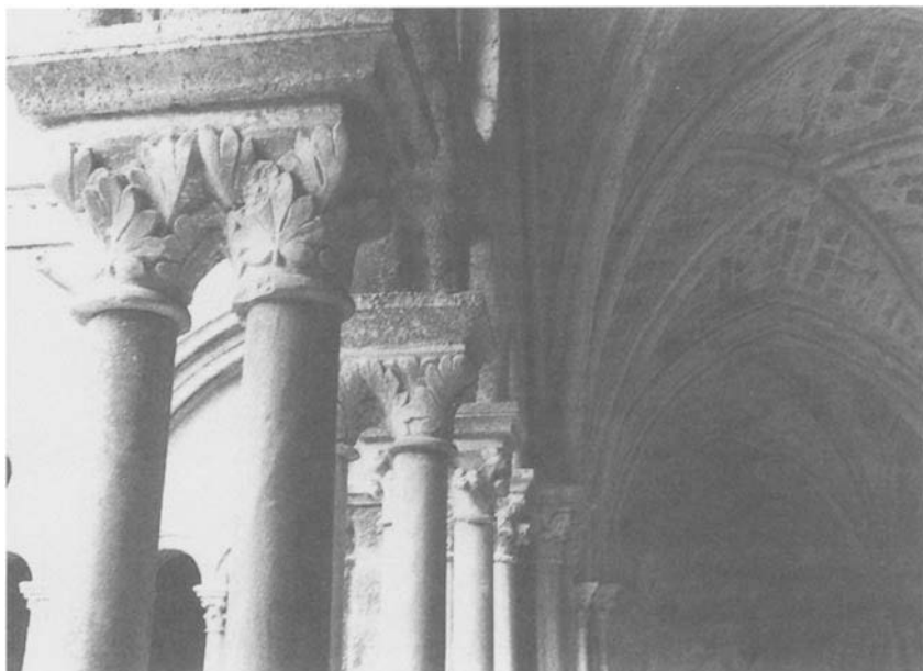
Figure 10. Fontfroide, cloister capitals.
