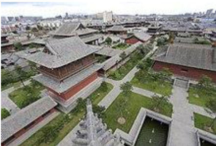
Aerial view of Huayan temple, Datong
