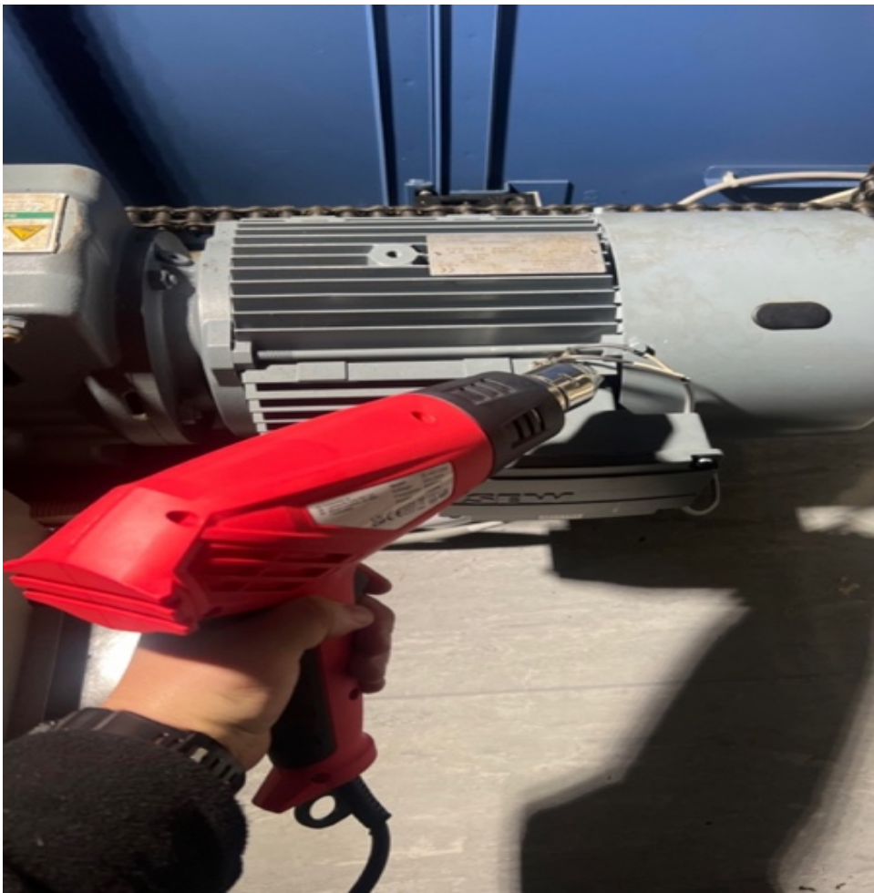
Heat Gun Test. Heating Motor Sensor to 100°C
