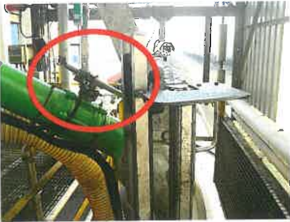
Figure 8. This illustrates a \frac{1}{4} turn ball valve, with a limit pack. This must be in the open position before loading can commence, if this valve is left closed the meter head will display a message highlighting this.
