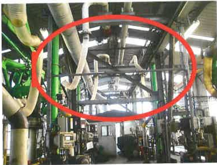
Figure 14. Illustrating the vapour recovery system on the Rail stand. It shows the vapour tubes from each arm piped into hardlines that go through flame arrestors, before being vented to atmosphere via a stack.
