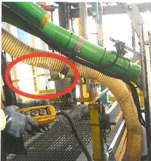
Figure 17. Illustrating a control pad for the loading arms.
