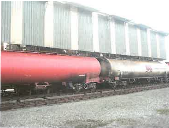
Figure 16. This shows the Western side of the rail stand and the 9 windows it has. These windows could be replaced with a clearer material to enable natural lighting into the Stand, or they could have sections cut out to again allow light in. This would reduce the energy consumption on the Rail stand drastically. Boyle G states "Natural lighting is more powerful than artificial lighting."
