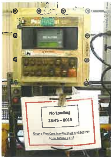
Figure 4. This shows one of the batch controllers on the Rail stand. This is where an Operator must manually input an index number, Rail car number and can input number pins to display flow rates, dye ratios and dye totalizers.
