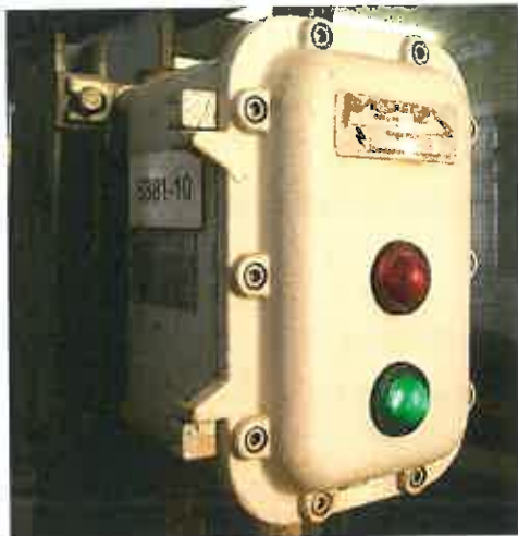
Figure 10. Shows the lighting system that is used by operators, this is a permissive system to prevent filling cars if the right sequence hasn't been followed. This lighting system also lets operators know whether they have a correct earthing on a Rail car, again without a green light no loading can take place.
