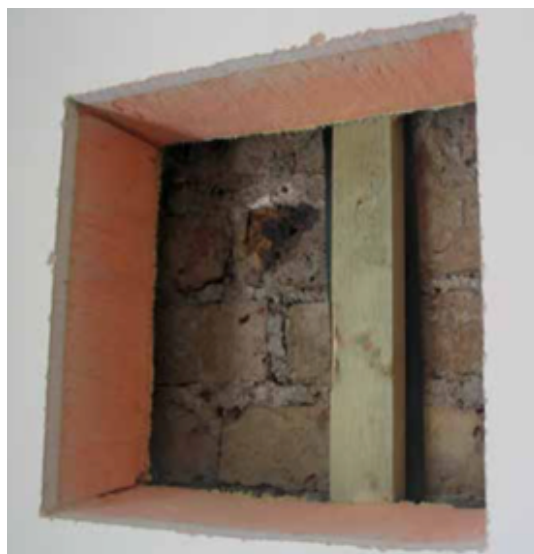
Figure 8: Internal insulation for solid wall
