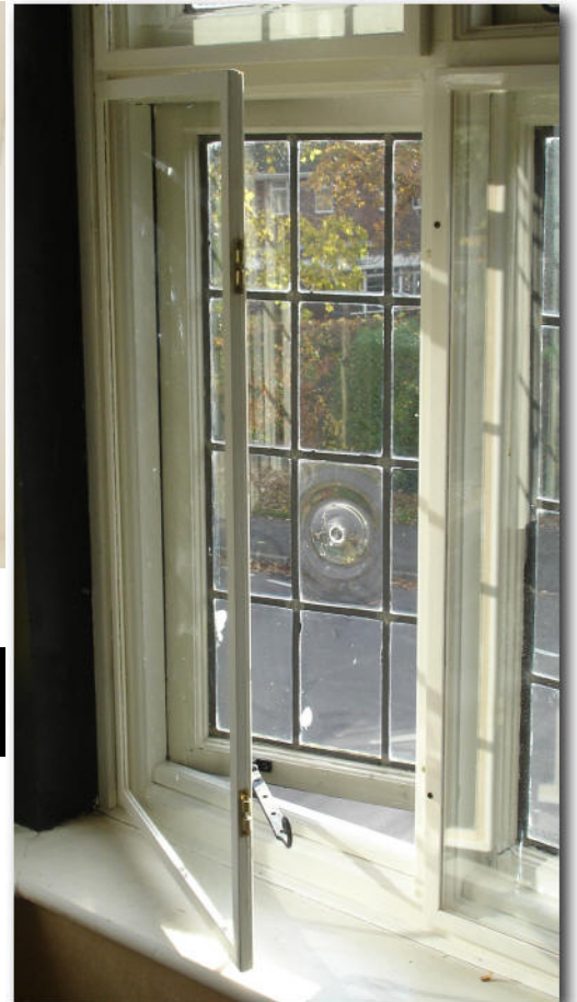
Figure 10.1. Frame System for Secondary Windows
