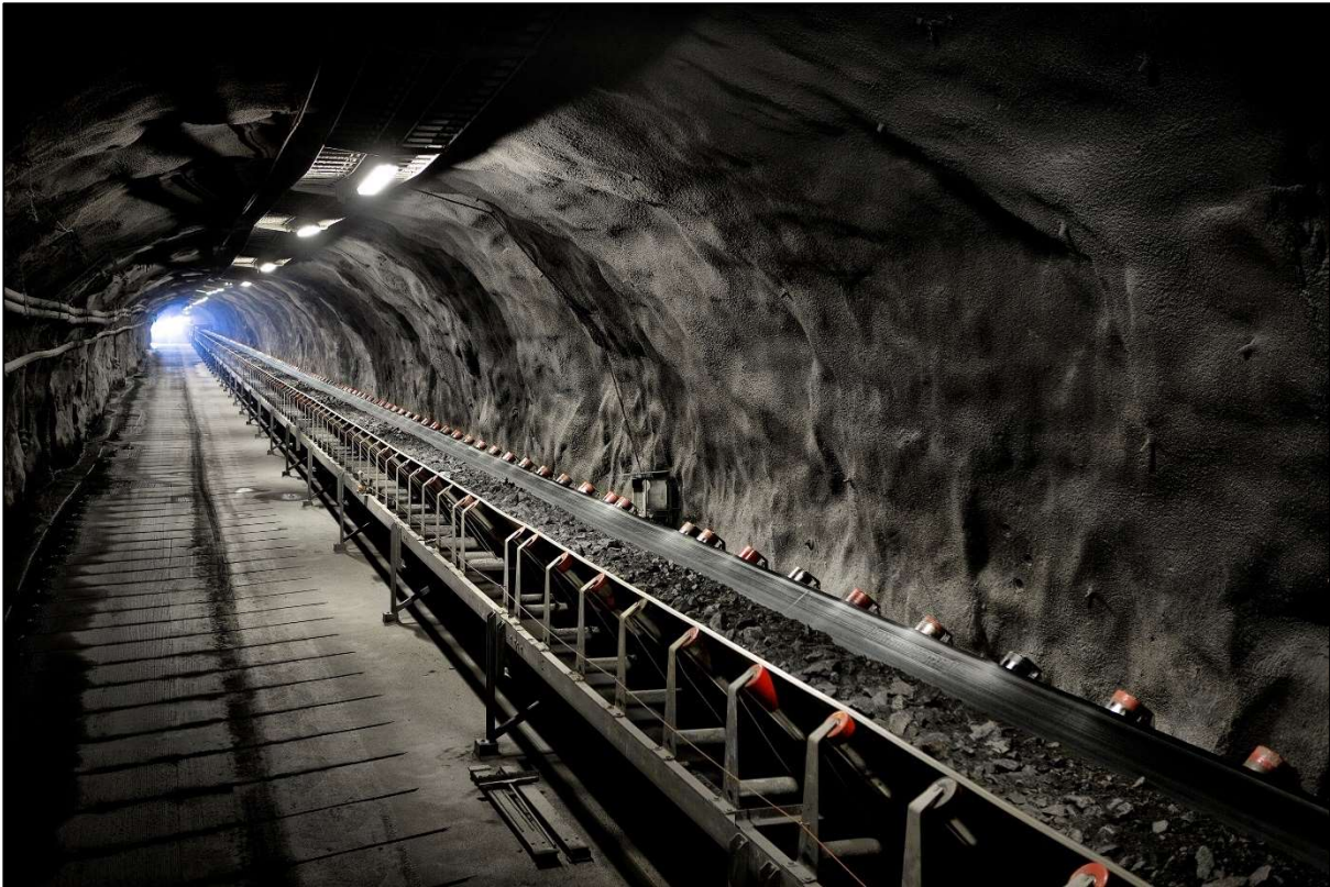
Figure 3 - Example of an Underground Conveyor in Kiruna, Sweden, courtesy of (Magazine, 2017)
