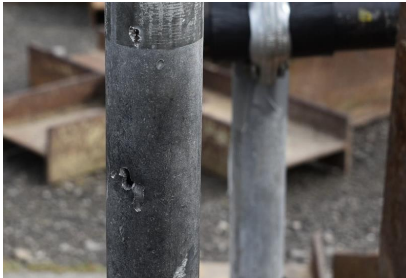
Figure 3 Fragmentation damaged pole
