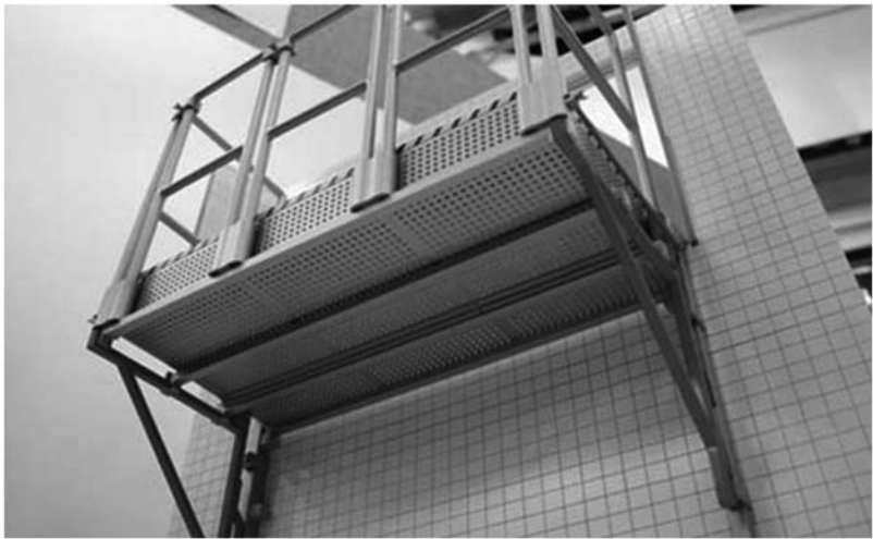
Figure 6.17 Underneath of RDP.
