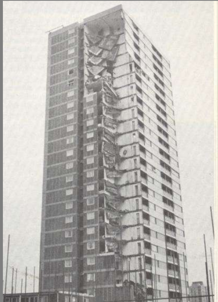
Ronan Point collapse 1968. Tide Turns
