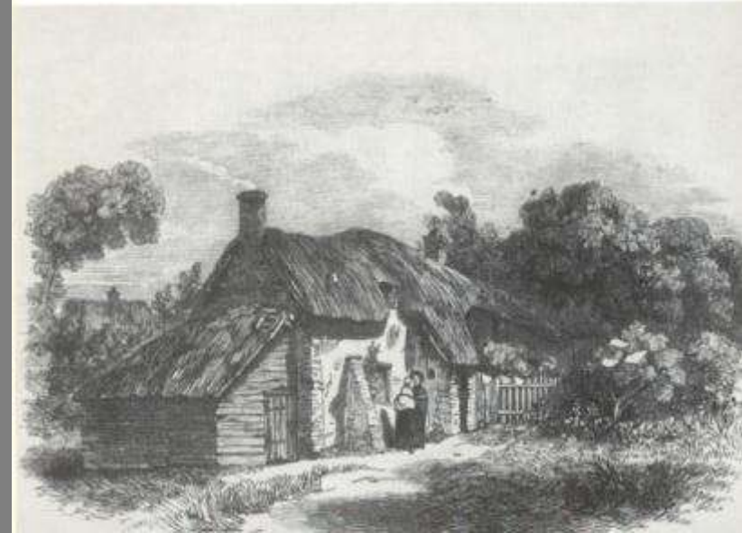
Rural decay: labourer's cottage near Blandford, 1846. The picturesque setting distracts attention from the decrepit roof (Illustrated London News)
