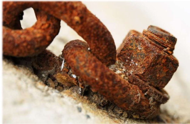
Image of a stud, nut and chain experiencing corrosion ( ExperimentosFaciles, 2016 )
