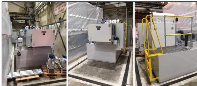
Figure 38: Oberlin Filter Placement
