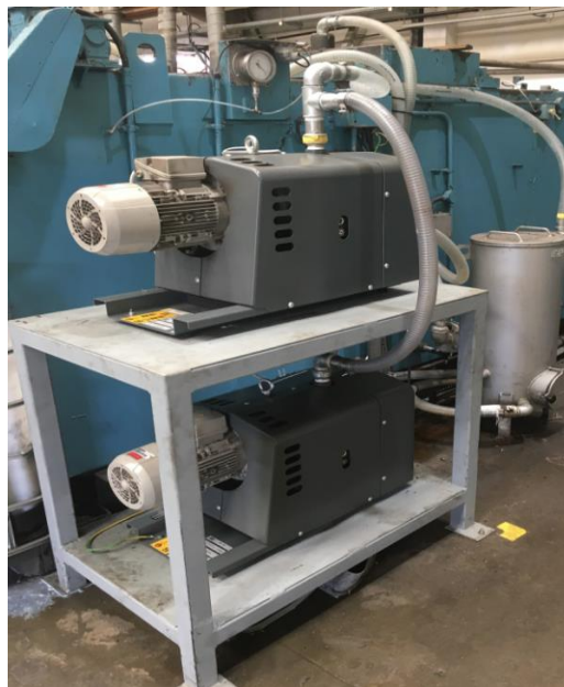
Figure 29: Controlgear Vacuum System Installation and Trial
