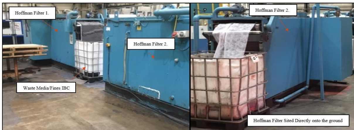
Figure 22: Hoffman Filters Prior to Drip Tray Installation
