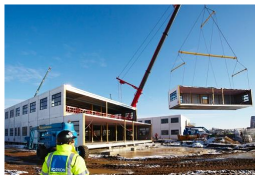
Figure 7 – Offsite Prefabrication (Designing Buildings Wiki, 2022)
