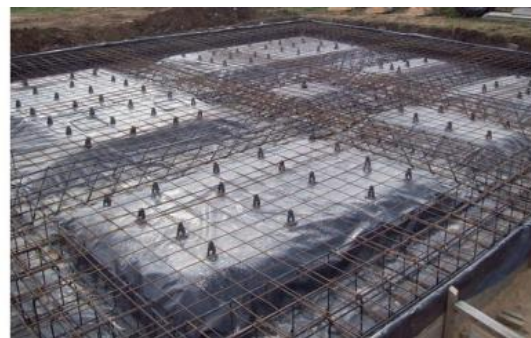
Figure 3 – Raft Foundation (LABC, 2018)
