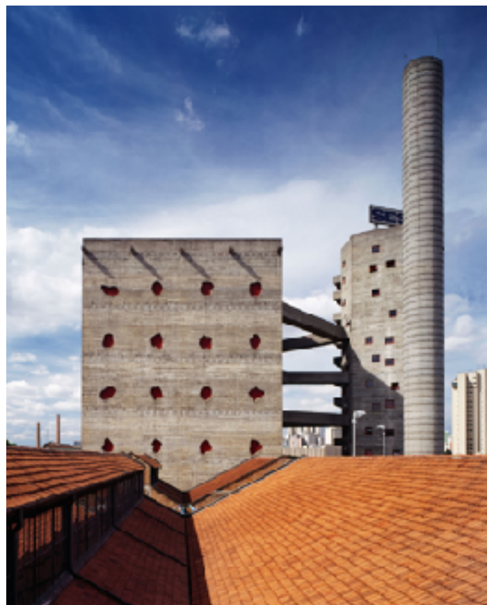
Figure 7: View from roof of old drum factory, (Impiraressa, 2015).
