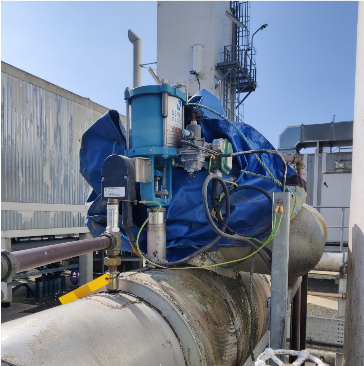
Figure 5 BOC oxygen valve
