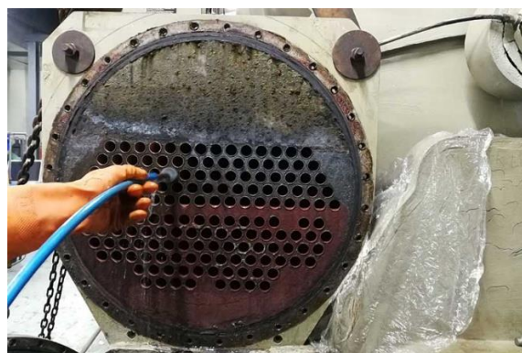
Figure 5: Image showing mechanical cleaning. (Baron Blakeslee)
