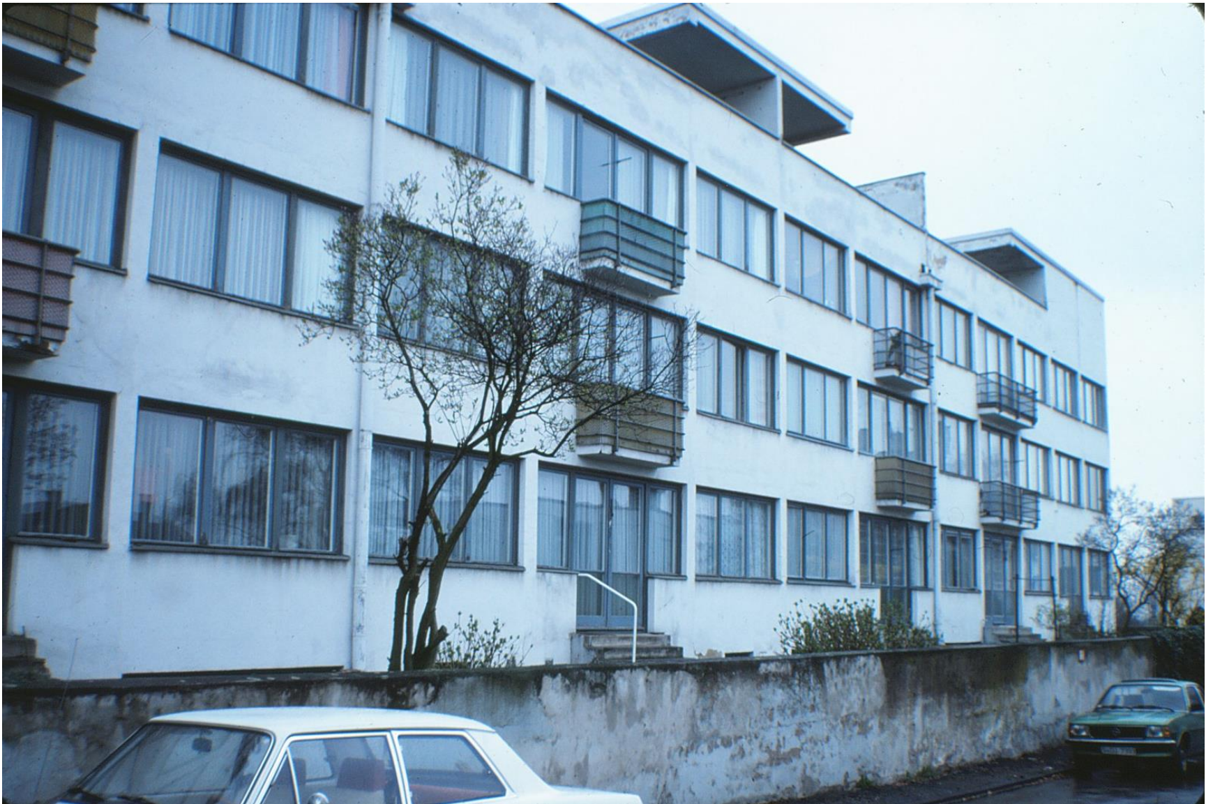
Weissenhof Apartment House, Stuttgart – 1926-27
