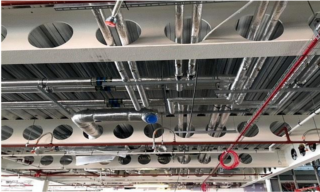
Figure 3.5: Castellated Beams (Cellbeam 2025)
