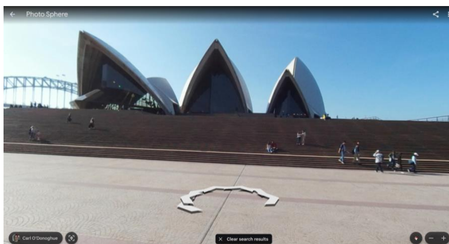
Figure 4.5: Sydney Opera House (Google Earth)
