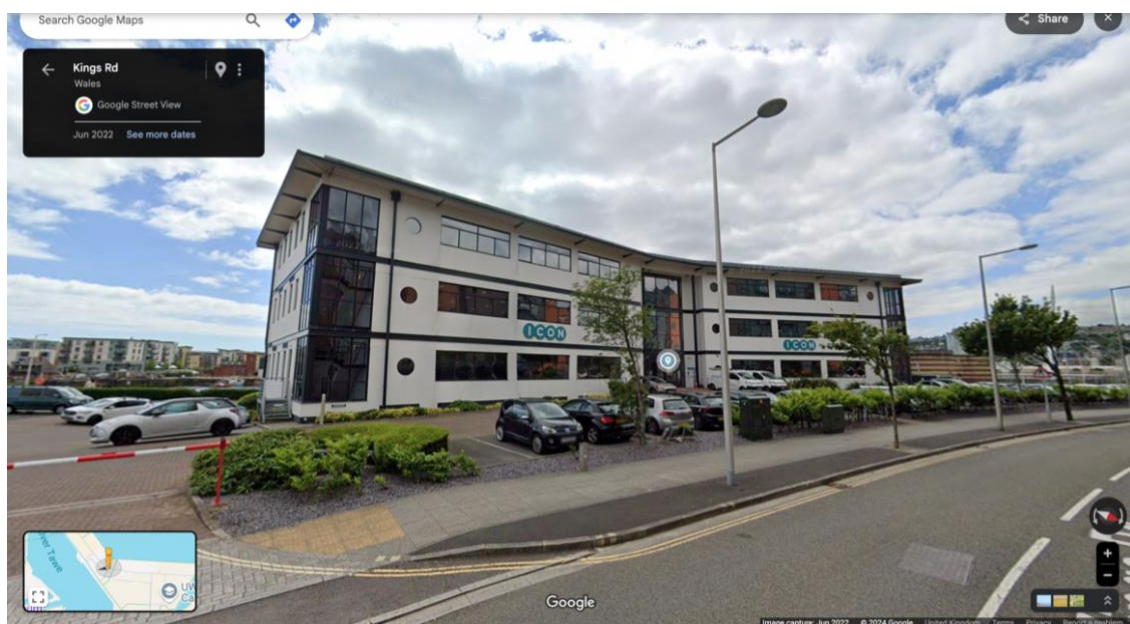
Figure C6: ICON Building on Kings Street
