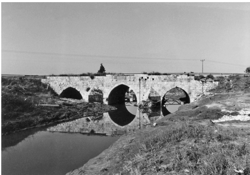
Fig. 5: Jisr Jindas view of southeast side of bridge with cutwaters
