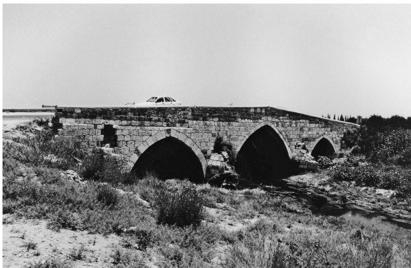
Fig. 9: Bridge at Yibna showing cutwaters
