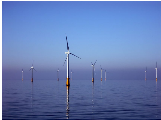
Figure 1: An offshore wind turbine site
