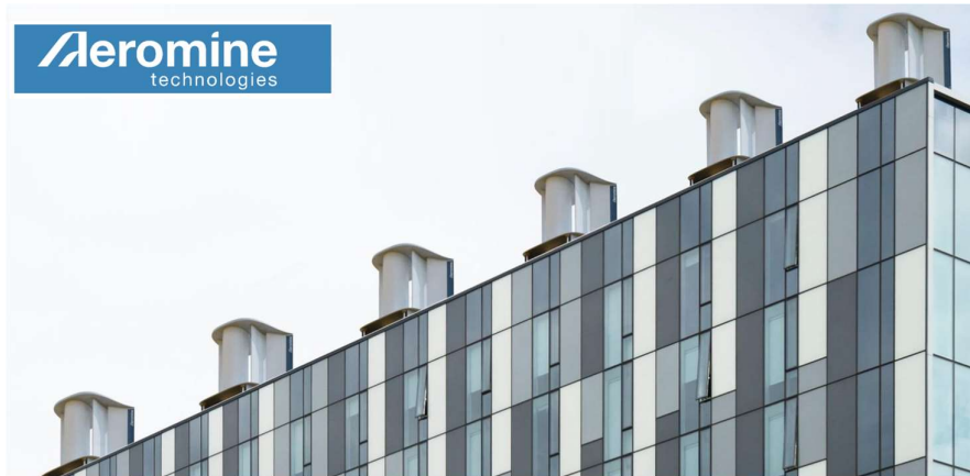
Figure 59 Aeromine Turbines on Roof of Building (Aeromine, 2024)
