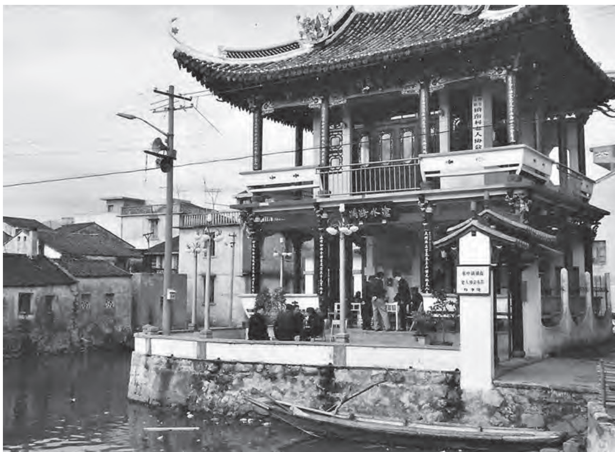
Figure 3.7. Old People's Pavilion in Yongchang Township, Longwan District, 1993. Photo by the author.
