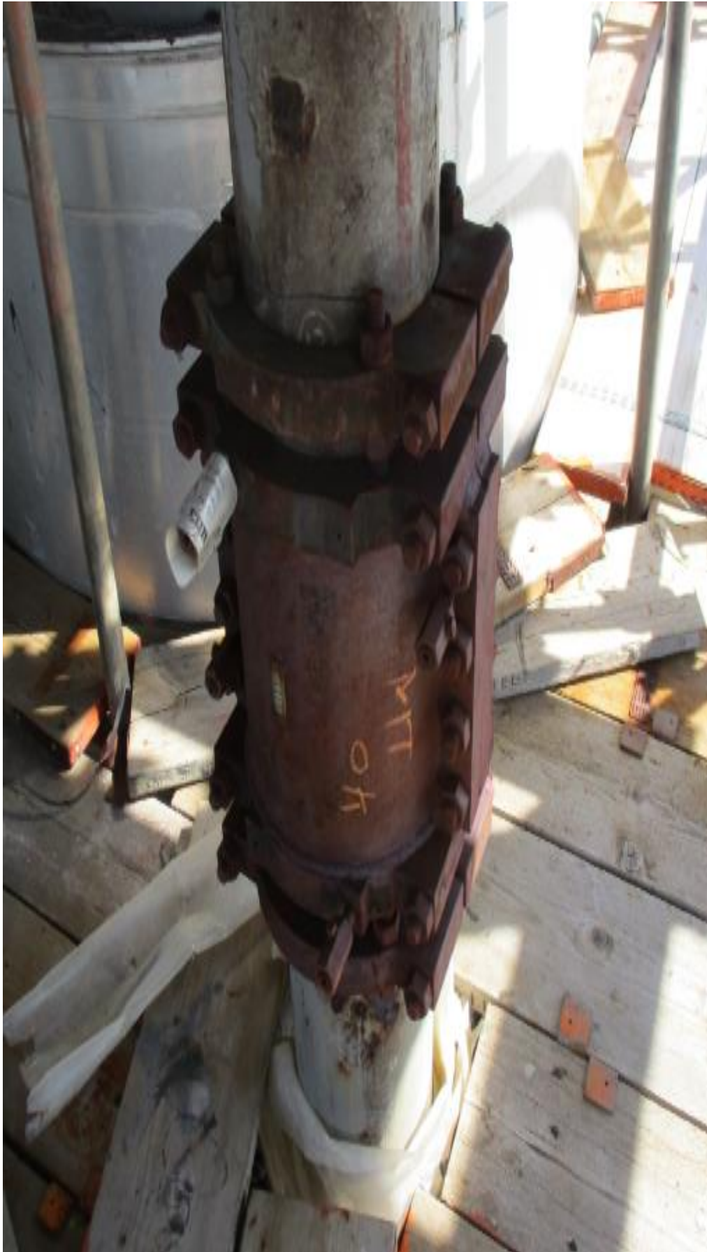
Figure 11 Clamp installed at location 12 of IAN (Clamp No. T26131)
