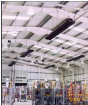
Individual gas-fired radiant-tube heaters in a postal depot. These heaters are linked to external flues. (Picture courtesy of Ambirad Ltd.)
