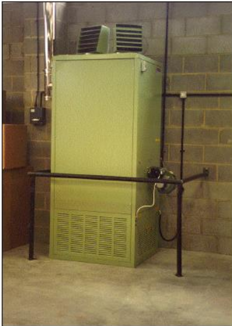
Free-standing warm air unit heater with a flue. (Picture courtesy of Powrmatic Ltd.)
