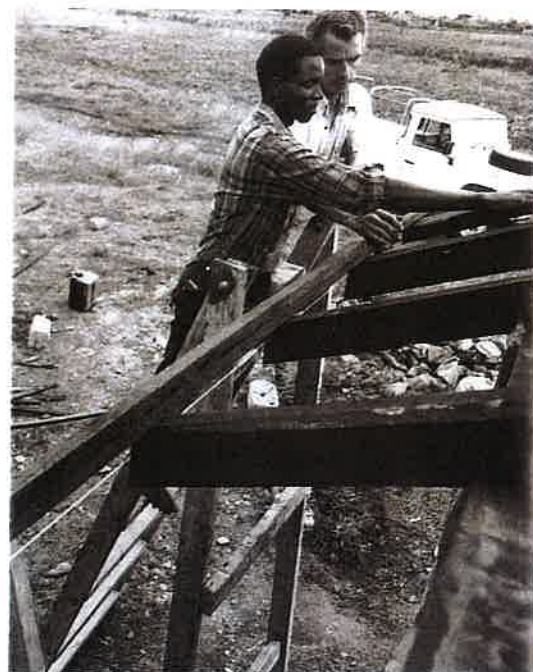
Building a teacher's house in Muka, Kenya
