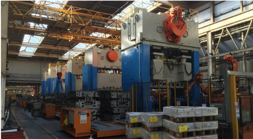
Figure 1: Picture of Line 3 after its installation
