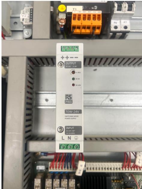
Fig.17 Power supply mounted
