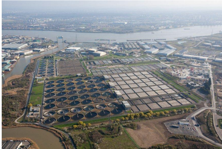
Figure 10 - Beckton Sewage Treatment Plant (Bell, 2017)
