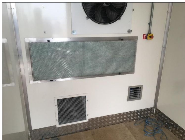
Figure 6 - Ventilation brackets and welded tread plate cladding
