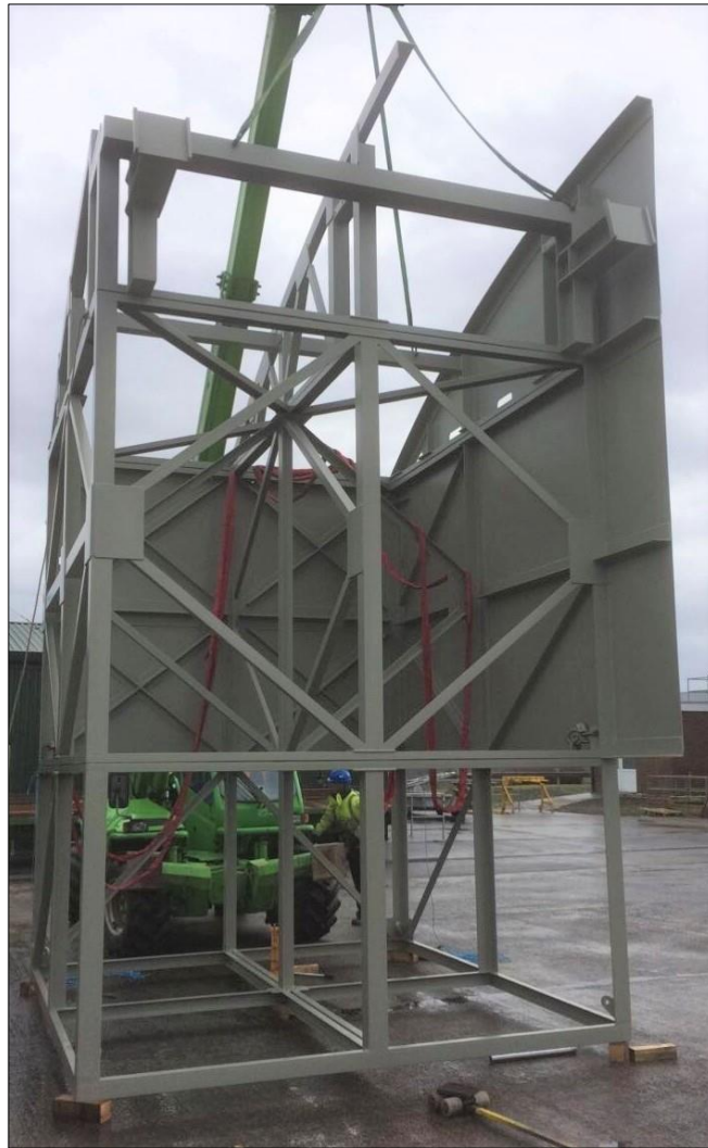
Figure 5 - Welded steel framework
