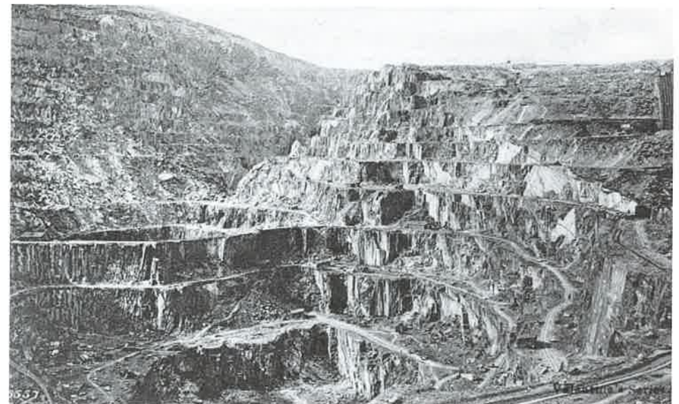
Penrhyn slate quarry
