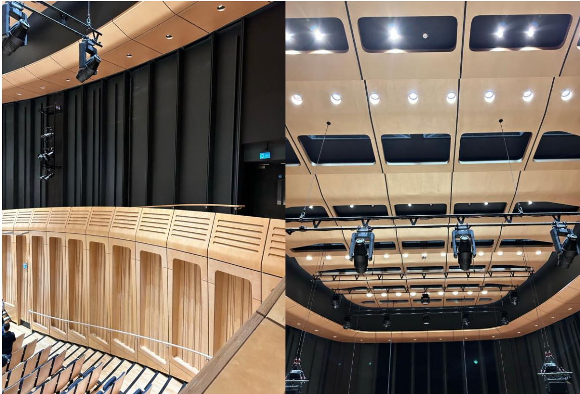
Figure 16: Dora Stoutzker Concert Hall using timber to enhance acoustic performance
