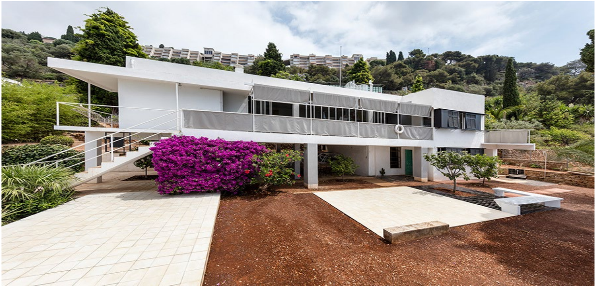
Figure 8: E. 1027. (Photo credit: Manuel Bougot)
