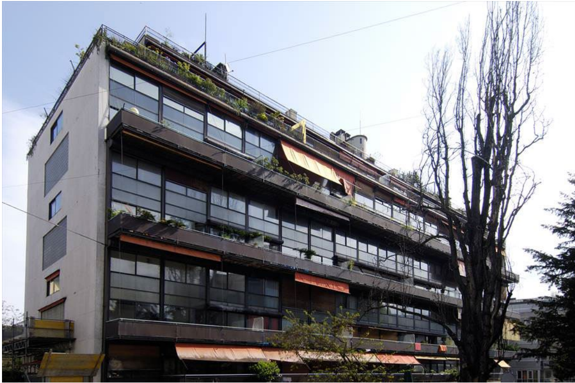
Figure 22: La Clarte Apartment Building, Geneva, after being adapted. (Photo credit: Eveline Perroud)
