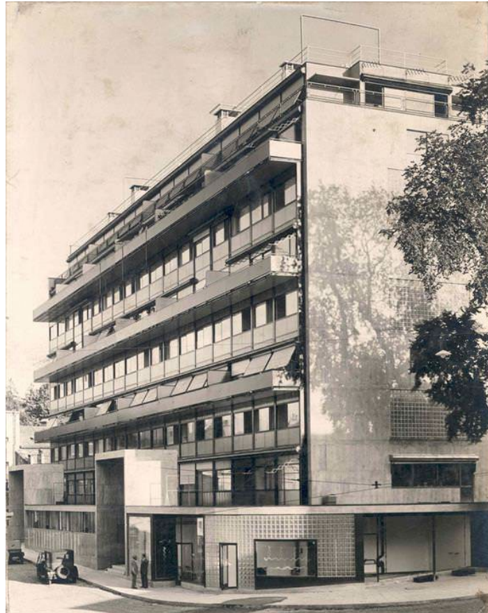
Figure 21: La Clarte Apartment Building, Geneva, before being adapted. (Photo credit: Fred Boissonnas)
