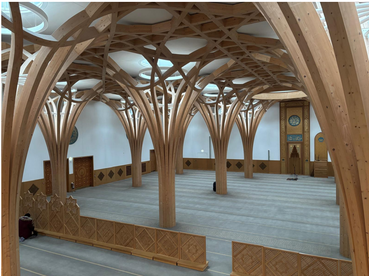
Figure 20: Shows the "Tree" columns which is made with glulam (Credit: William Wilson)
