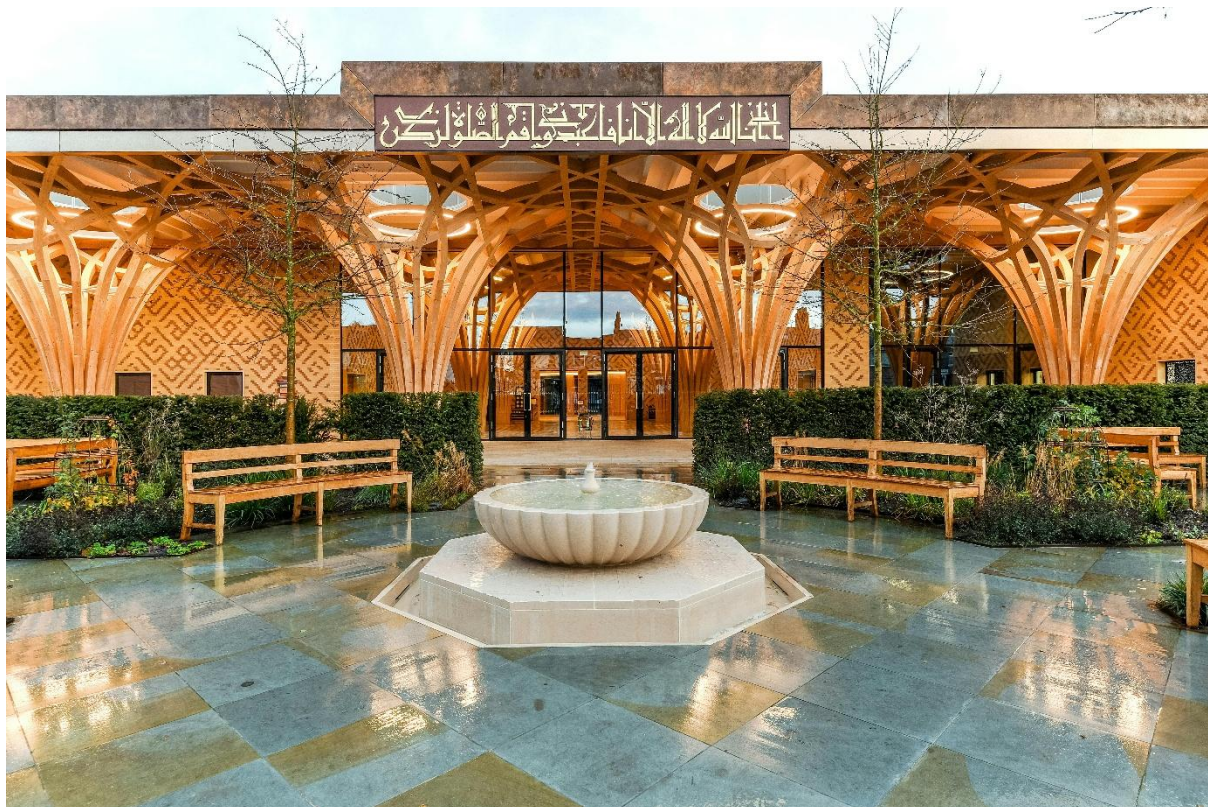
Figure 24: View of the main entrance showing the brick cladding and the "trees" columns (Credit: Amelia Hallsworth)
