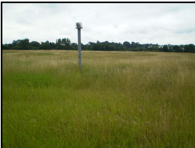
Photograph 7 - On Site Vent Stacks
