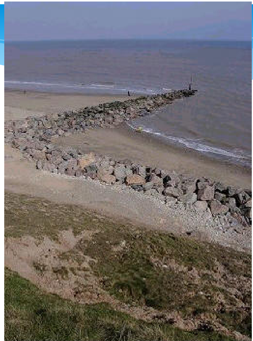
A stone groyne at Mapplelton, Holderness, in Yorkshire. Rip rap protects the cliff in the foreground. a small beach has built up to the north of the groyne.
