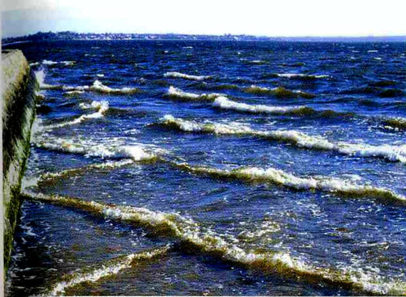
Figure 17.13 Reflection of breaking waves at the vertical face of a seawall giving rise to a criss-cross wave pattern.
